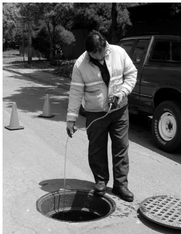
A member of the collection crew checks for sewer gas.
