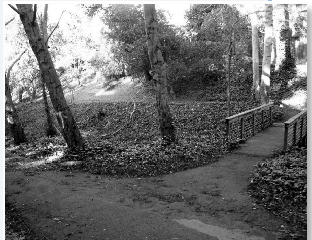
Sewer lines along Baxter Creek were recently sliplined to protect the creek from possible sewer failure.
